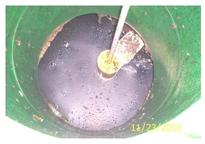
Remove the filter from the baffle. Use a small hoe or rake or pull it out by hand. Wear disposable gloves for protection.
