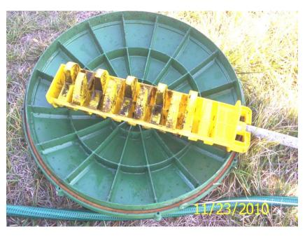
Once all debris has been removed re-install the filter properly. There may be an arrow on the filter for proper installation.
